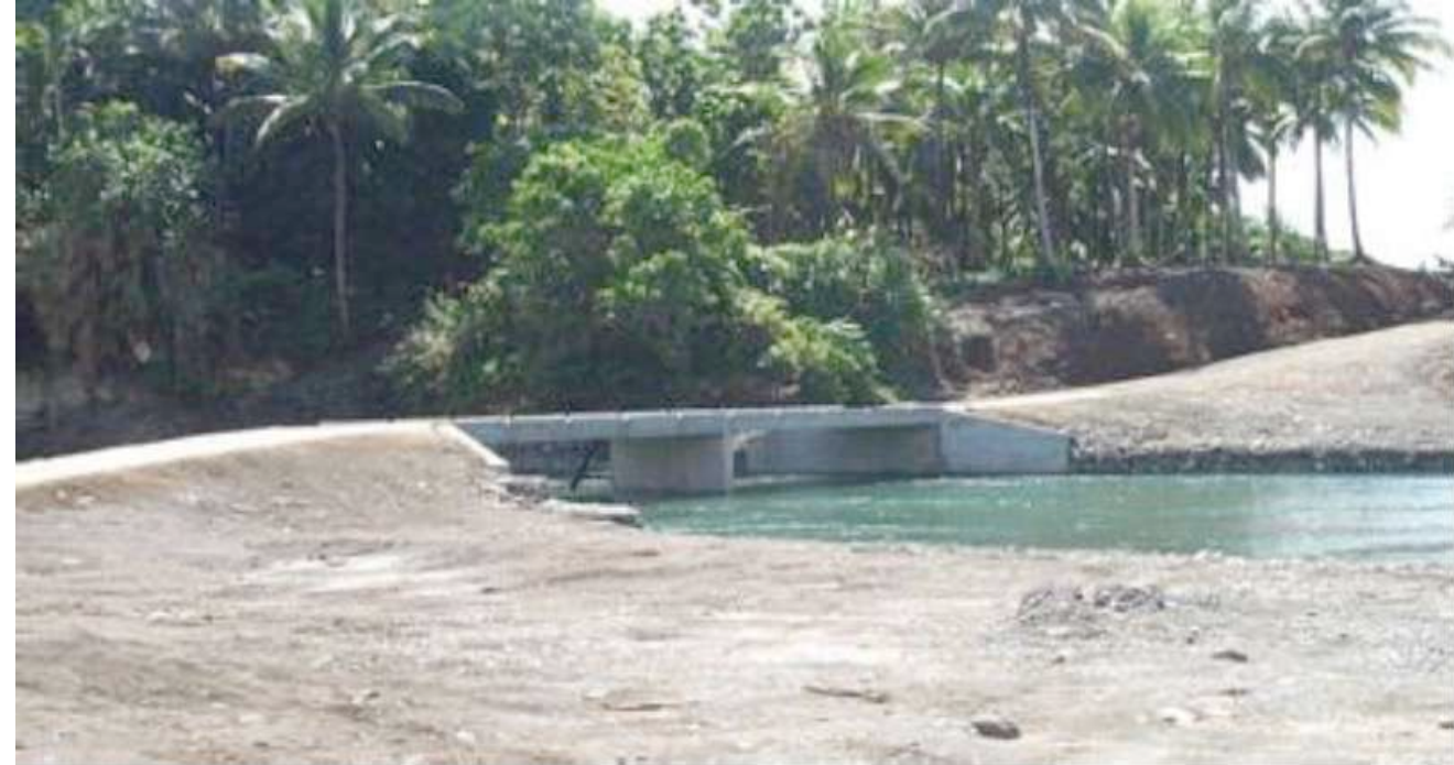
Replacing bridges with less brittle river-crossing sills (AFD in Vanuatu)
